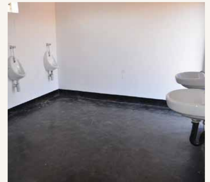
New toilet facilities at Madima Primary School
